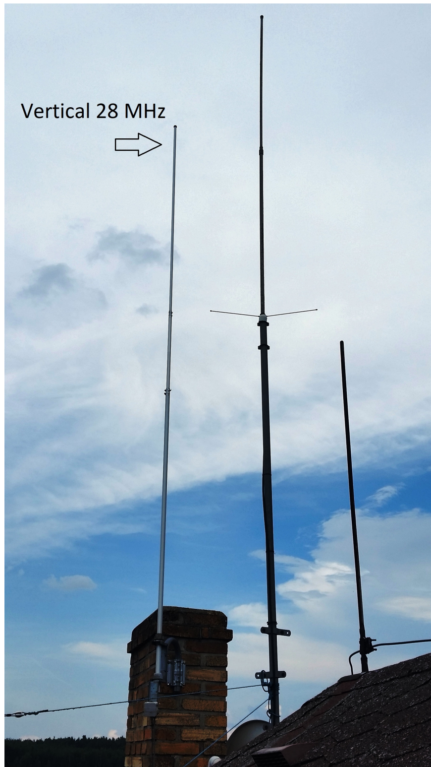
Figure 3.9: Half wave vertical antenna used for remote transmission
